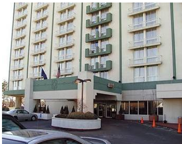
Doubletree Hotel JFK Airport
